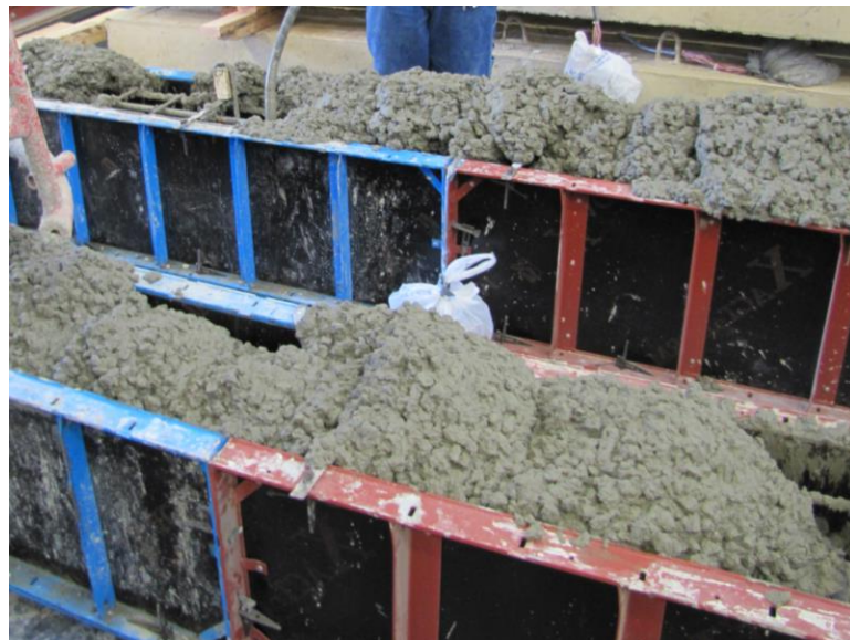
Figure 4.12: Casting of Beam Splice Specimens
