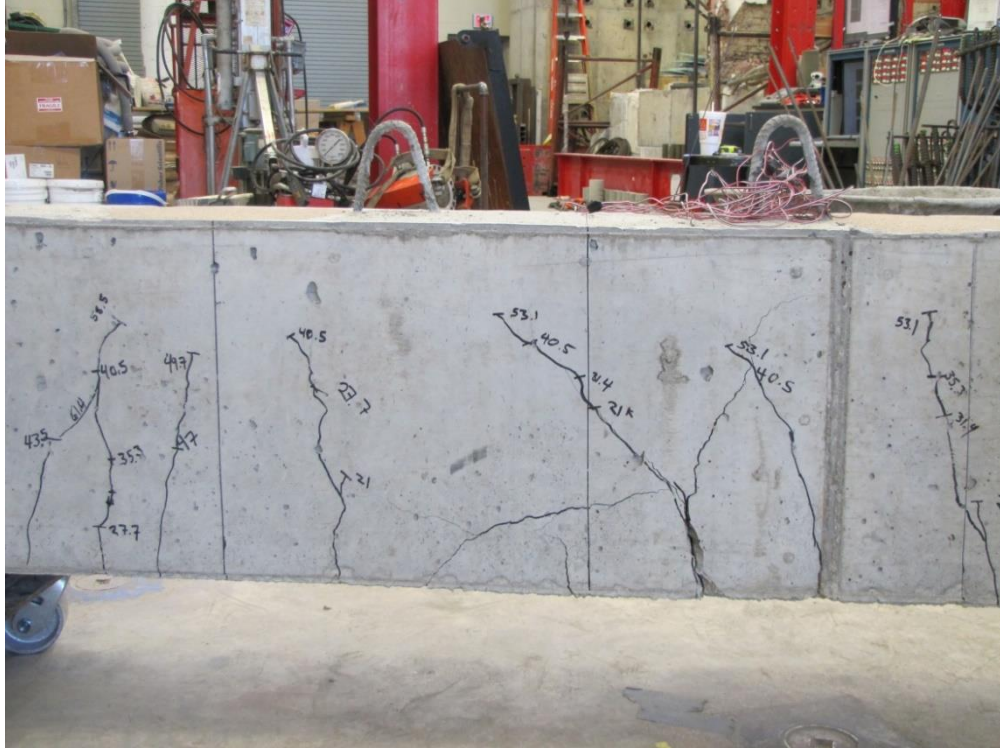
Figure C.3: Side View of VAC-2
