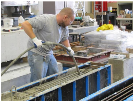
(c) Concrete consolidation
