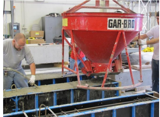
(b) Concrete placement
