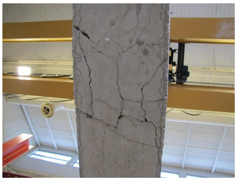
Figure 5.14: Beam Splice Specimen Bottom View at Failure (RAC50-1)
