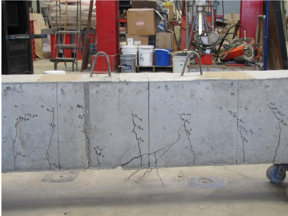
Figure C.1: Side View of VAC-1
