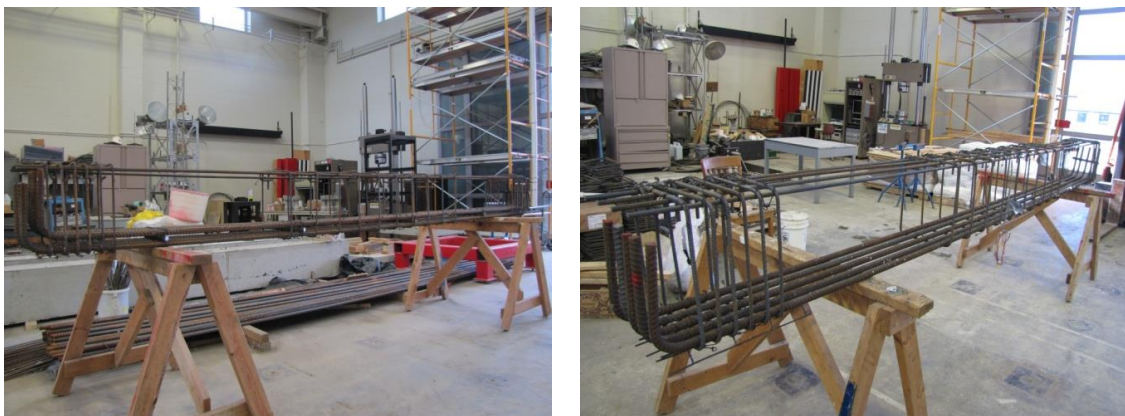
Figure 4.3: Reinforcing Cage Assembly
