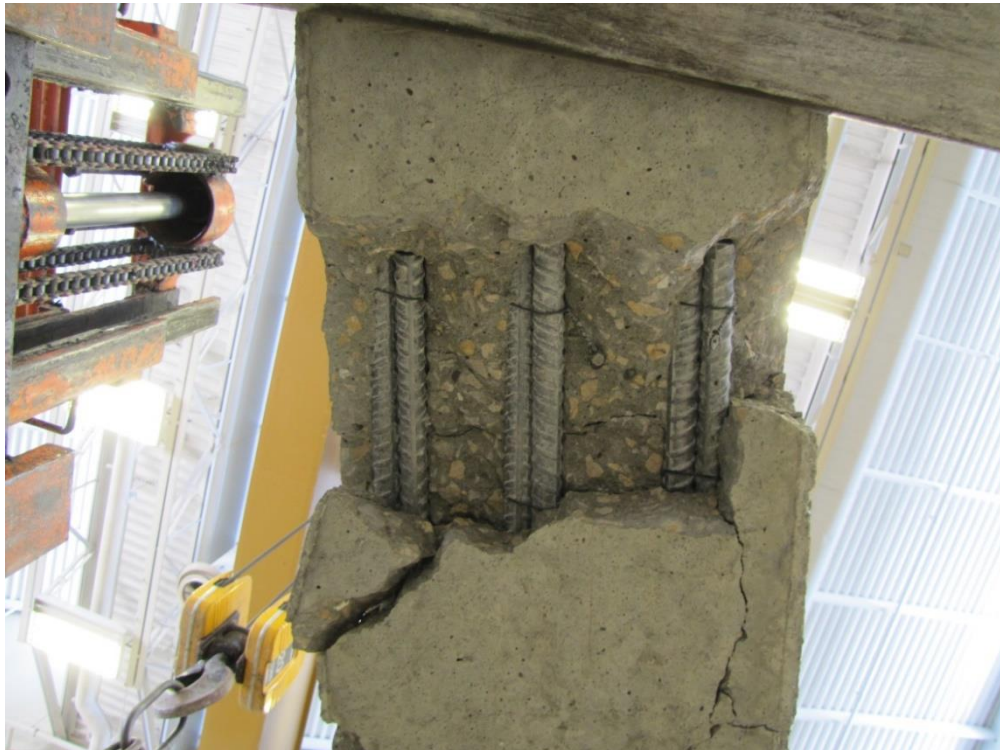
Figure C.6: Bottom View of VAC-3
