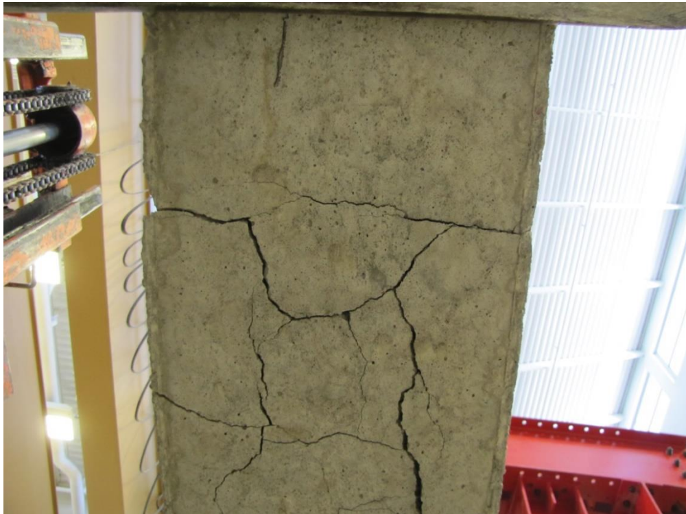
Figure C.4: Bottom View of VAC-2
