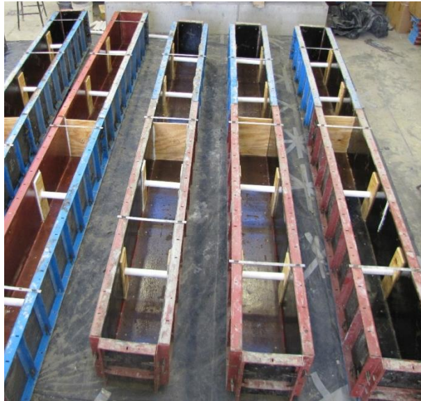
Figure 5.1: Concrete Beam Molds with PVC Conduits
